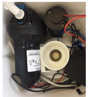
15. Replace rinse pump & control box
